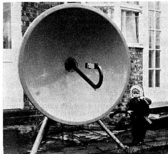
"Big 3cm dish, small 60cm daughter." G3WJG's 10GHz dish and mount as used on the recent GC expedition
